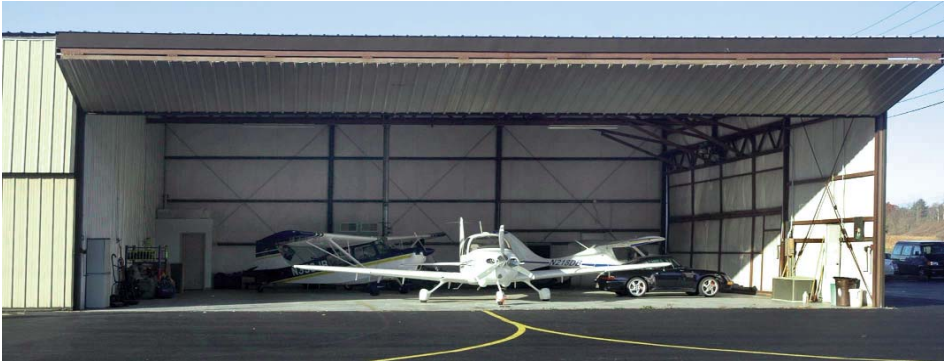
Wings plans to build five hangars such as this 65' wide x 62' deep x 23'6" high insulated unit. Each unit can hold up to four single-engine planes or three twins or one turboprop or one business jet or other combinations.
