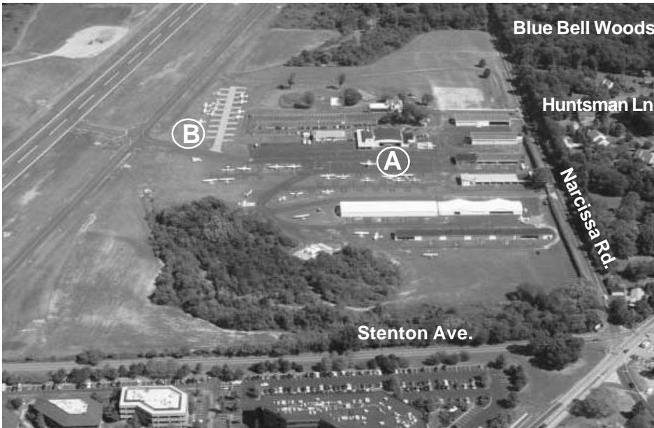
Wings plans to move the parking area for visiting turbine aircraft down the hill from the terminal area (A) and next to the taxiway (B). It will improve quality of life for neighbors.
