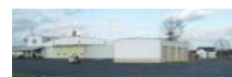
Wings Field's four bay snow removal equipment building will be located near the entrance of the field, next to the administration building (left) and the maintenance hangar (center). The small building on the right is the headquarters for the PennStar medevac unit.
