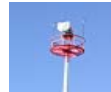
Most airports are equipped with rotating light beacons to make them easy to locate at night. At most civilian airports the rotating beacon alternately flashes green and white. Military airfields beacons like Willow Grove and McGuire flash white, white, green. They operate from dusk to dawn or when the weather has gone to instrument meteorological conditions.
