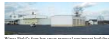
Wings Field's four bay snow removal equipment building will be located near the entrance of the field, next to the administration building (left) and the maintenance hangar (center). The small building on the right is the headquarters for the PennStar medevac unit.
